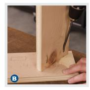
B Use #2 driver bit to drive two 1 <sup>1</sup>/<sub>4</sub>" pocket-hole screws.
